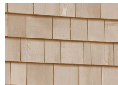
Wall Siding: Cedar Shingle Siding
