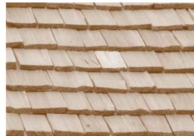
Roof: Heavy Treated Hand-Split Cedar Shake Shingles
